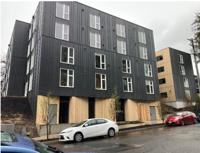
The first Shortstack project which recently completed construction.
