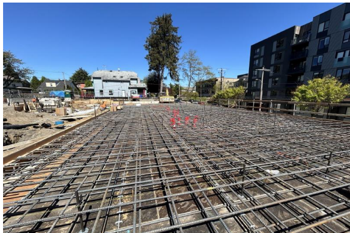
Concrete foundation ready to be poured for the first project.
